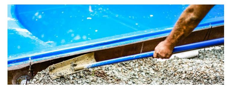
Once plumbing is done, and the pool shell is set and leveled, it's time to **fill the pool with water** and **backfill the perimeter with gravel**.
