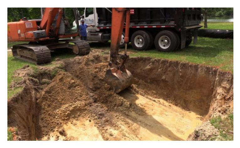
The first thing we'll do is "paint" the pool on the ground and use a laser level to establish how high to set the pool in the yard. This tells us how deep to dig. A dump truck will be moved close to the hole if needed before excavation begins.
