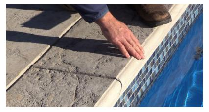
Once the pool's completely backfilled and inspected, our team can install coping around the rim of the pool shell and the pool patio. The patio crew may start work anywhere from a few days to two weeks after backfilling, depending on weather and inspection schedules. Patio construction usually takes between two and five days, depending on its size and the materials used.
