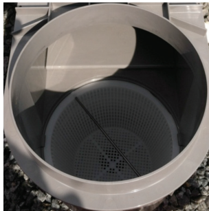
Skimmer basket (located in the skimmer box at the pool)
